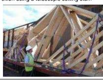
8. The crane will then lift the truss pack from the bed of the trailer. **NEVER** stand in the danger area where the trusses could potentially fall. Do not allow any others to enter the danger area.
